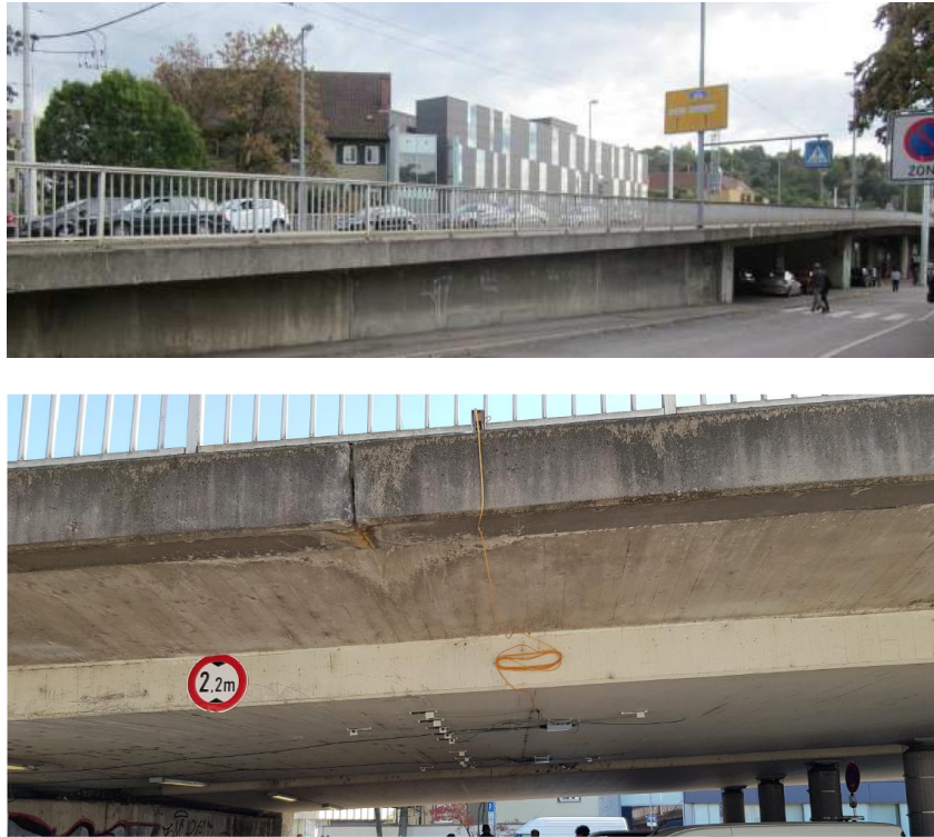
Fig. 16: View and instrumentation of the selected section of the Vogelsang bridge, Esslingen, Germany.
